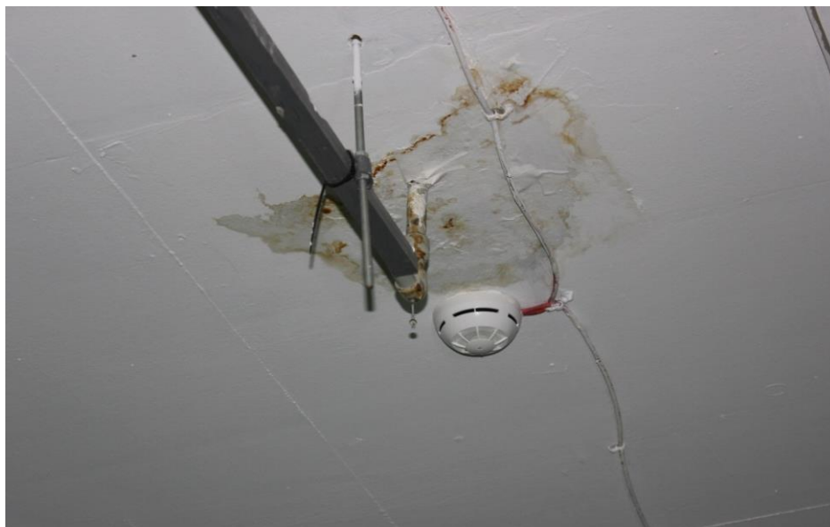
Photo 5: Depository in the current building
