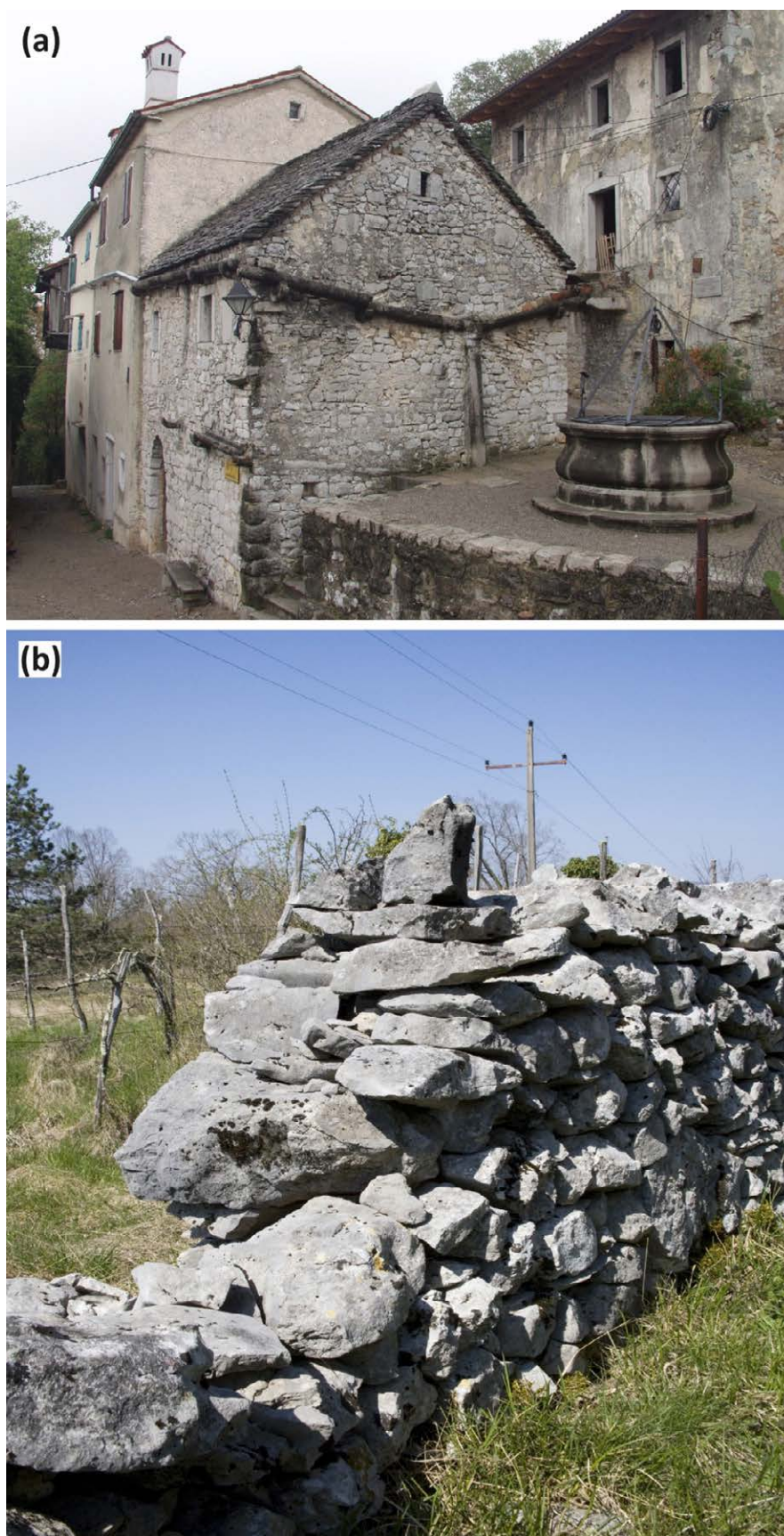
Figure 13. (a) Kras village Štanjel—examples of the traditional use of limestone in the Classical Karst: stone gutters, fountain, construction material, stone roofing, window frame and stairs (photo Valentin Benedik), (b) Archaeological site Debela Griža-Volčji Grad in Kras; dry-walled construction.
