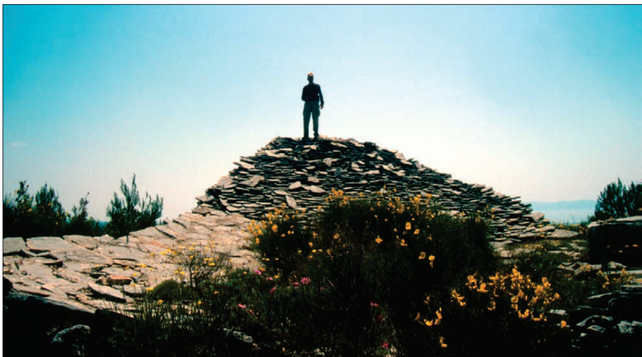
Figure 21: A 'naplov' can be several metres high; its surface can be some hundred square metres, island of Hvar, Croatia (Photo: B. Juvanec).
