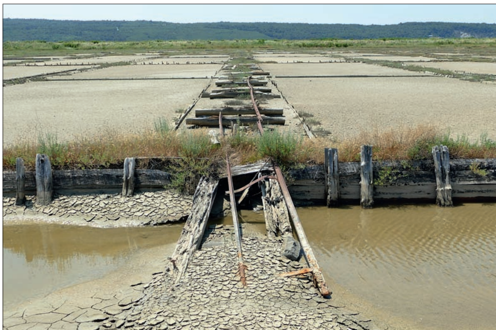
Figure 5: Lera South – abandoned salt crystallisation pools (S27).
