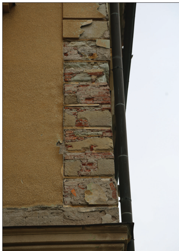
Figure 11: On one of the corners of the manor, older building elements processed by stonemasonry are used as a spoliation, 2022 (Photo: I. Sapač).
