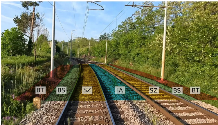
Fig. 2 Railway zones as defined in the floristic sampling: SZ (Sleeper Zone), BS (Ballast Shoulder), BT (Ballast Toe) and IA (Intertrack Area), adapted according to Sadeghi et al. (2016), Alabassi and Hussein (2021) and Guo et al. (2022). Two railway marking stones (left bottom and middle of picture) represent the defining starting and finishing points for the 100-m transect length
