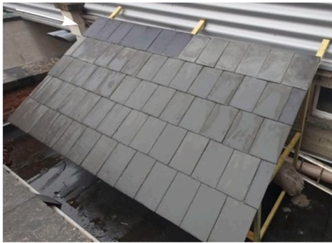
Fig. 13. AAM roofing tiles installed on a demonstration roof. The seven tiles in the top line (arrow) were treated with an additional coating not discussed in this manuscript.
