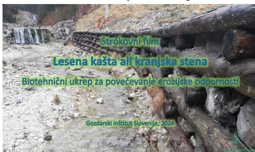
Figure 12: Wooden chest or Carniolian wall – a biotechnical measure for increasing erosion resistance (Saražin, 2024); https://youtu.be/btj_nt4FHUw
