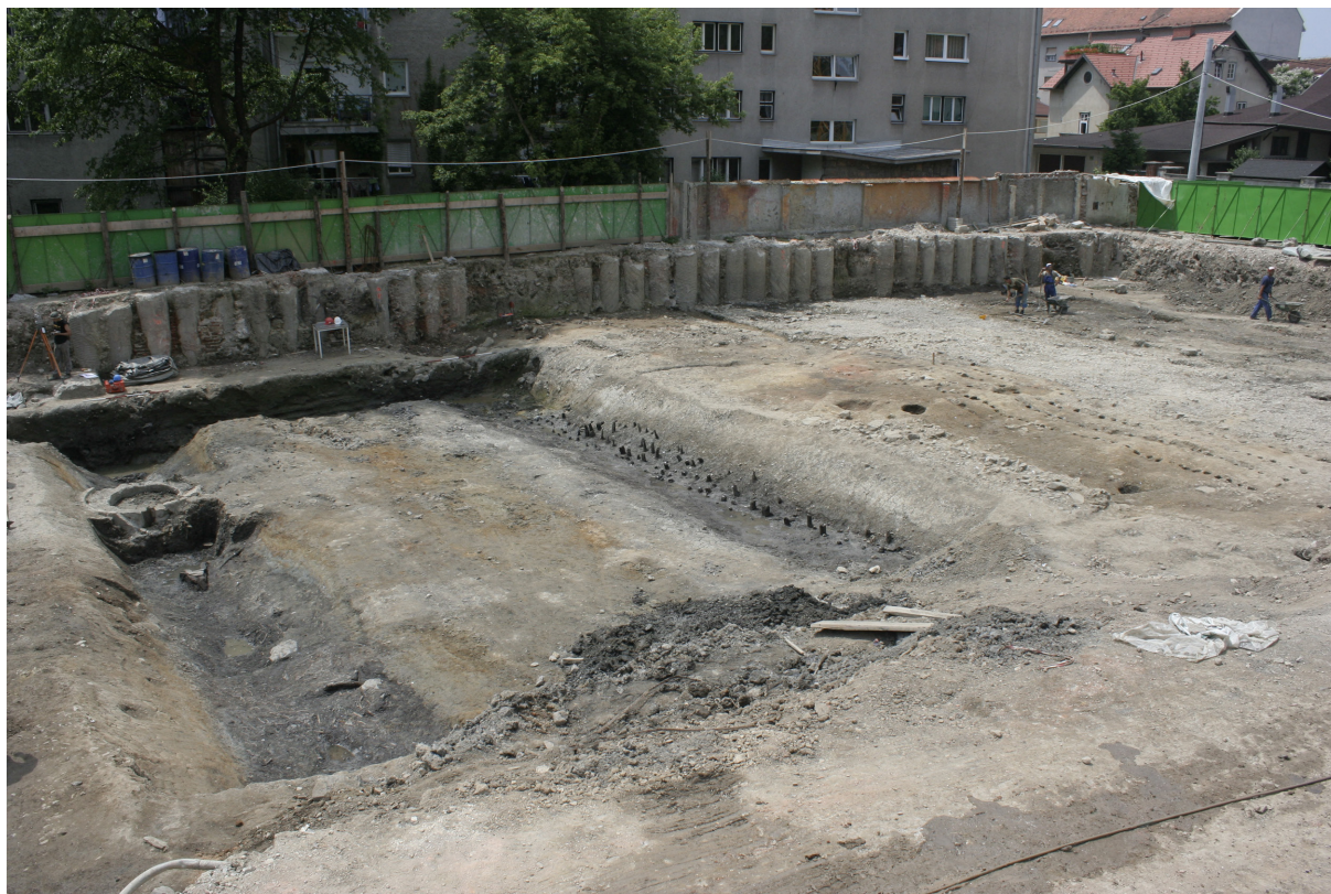
Fig. 10: The earlier fort on the right bank of the Ljubljanica in Ljubljana, from left to right: the two defensive ditches, lines of holes indicating the position of vertical beams in the already dismantled defensive wall, and via sagularis ; view to the west-southwest. Sl. 10: Starejši tabor na desnem bregu Ljubljanice: obrambna jarka, vrste lukenj, ki kažejo lego navpičnih lesenih kolov v že odstranjenem obzidju, in via sagularis ; z leve proti desni, pogled proti zahodu oziroma jugozahodu.
