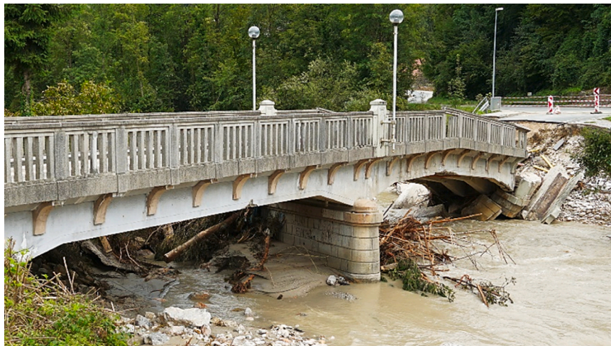
Fig. 1. Example of bridge collapse under scour in Slovenian flood in 2023.
