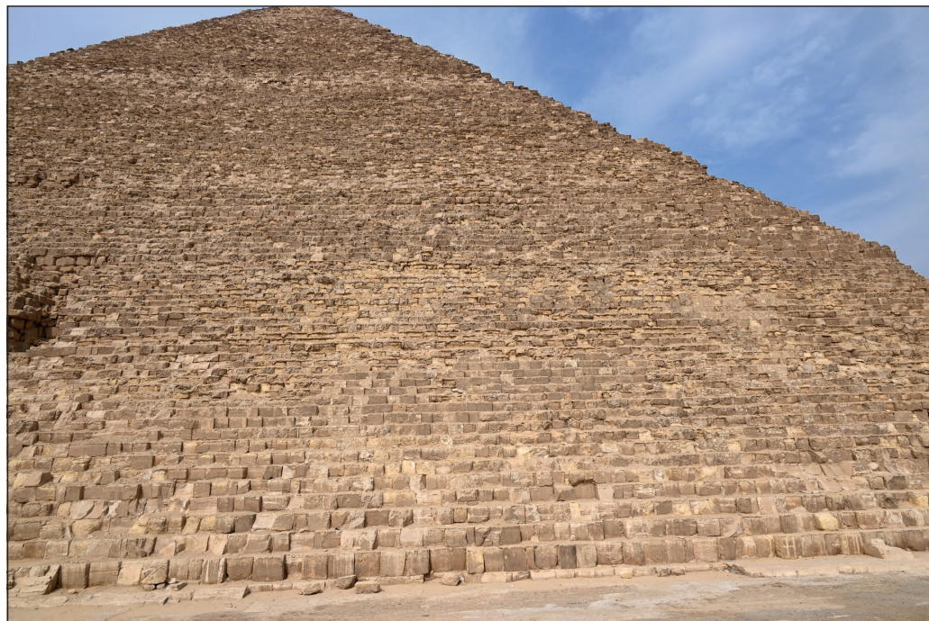
Figure 40: Stratification of the pyramid because of different rock.
