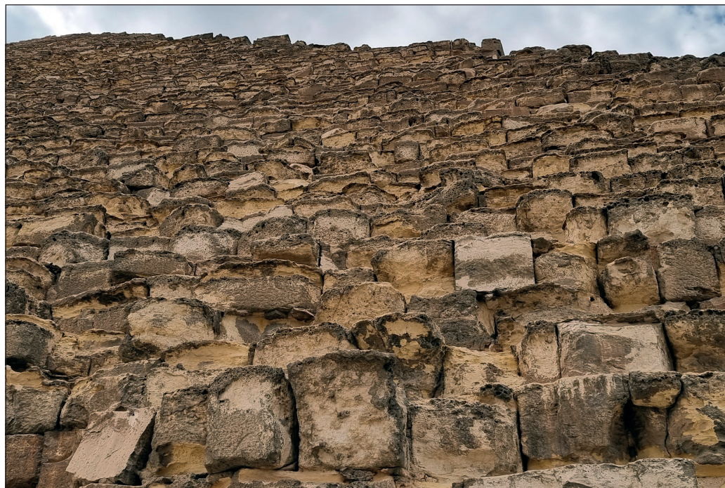
Figure 17: Eroded stone blocks. Width of view, lower part, is 12 m.
