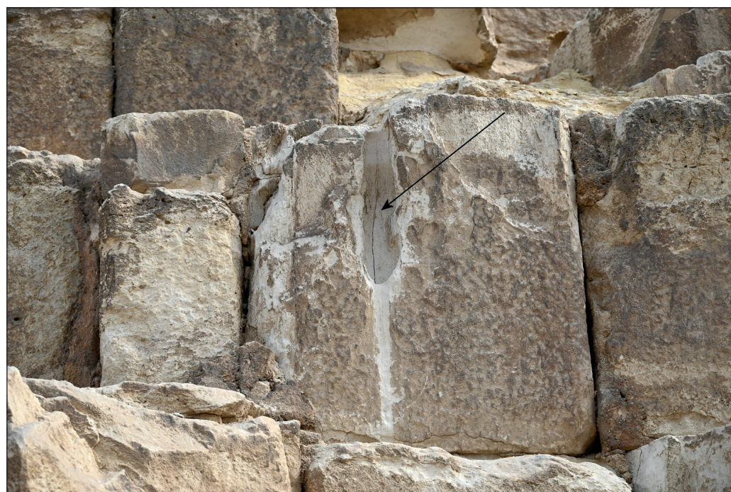
Figure 41: Wall channel. Width of view is 3.5 m.
