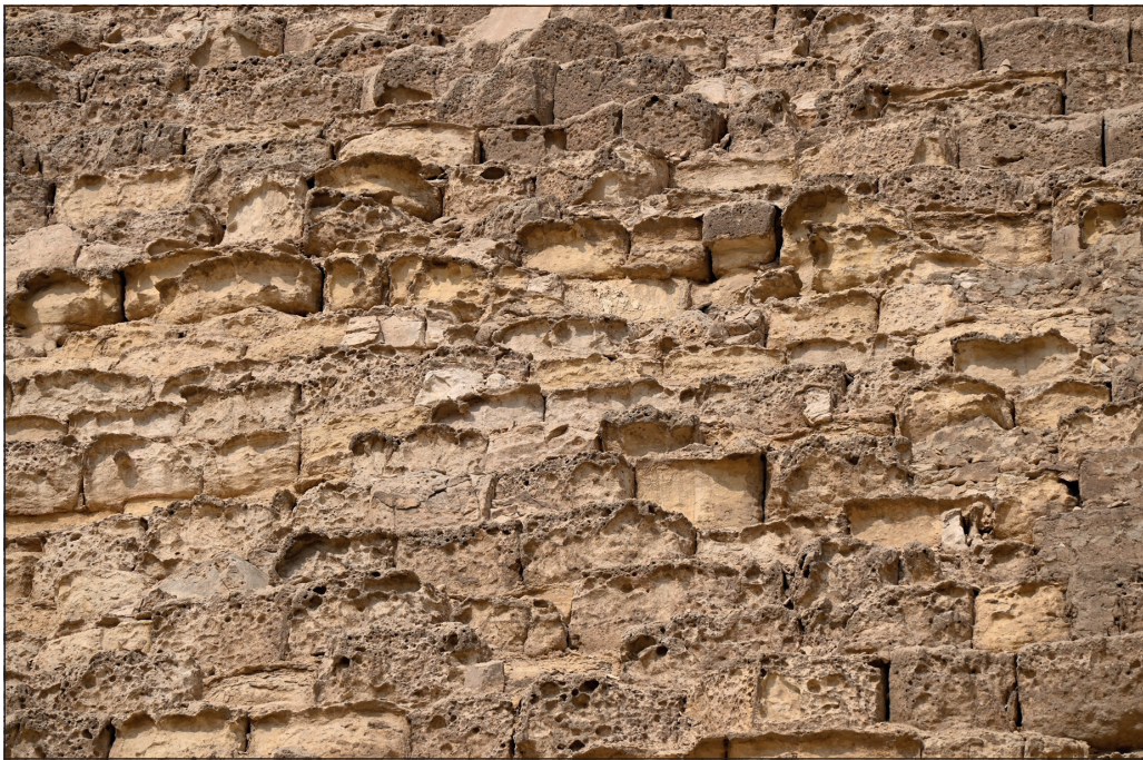
Figure 30: Wind-formed depressions. Width of view is 15 m.
