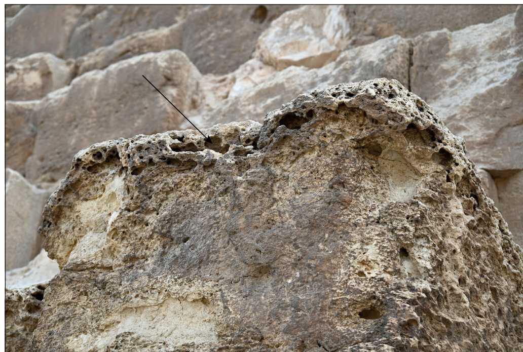
Figure 19: Cups and pits (arrow). Width of view is 1.5 m.
