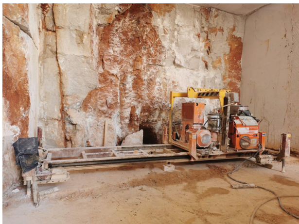
Figure 1: Fantini 70-RA-BU bank chainsaw machine in the Debela Griža quarry, Slovenia. Gallery width of 5.1 m and height of 4.0 m.
