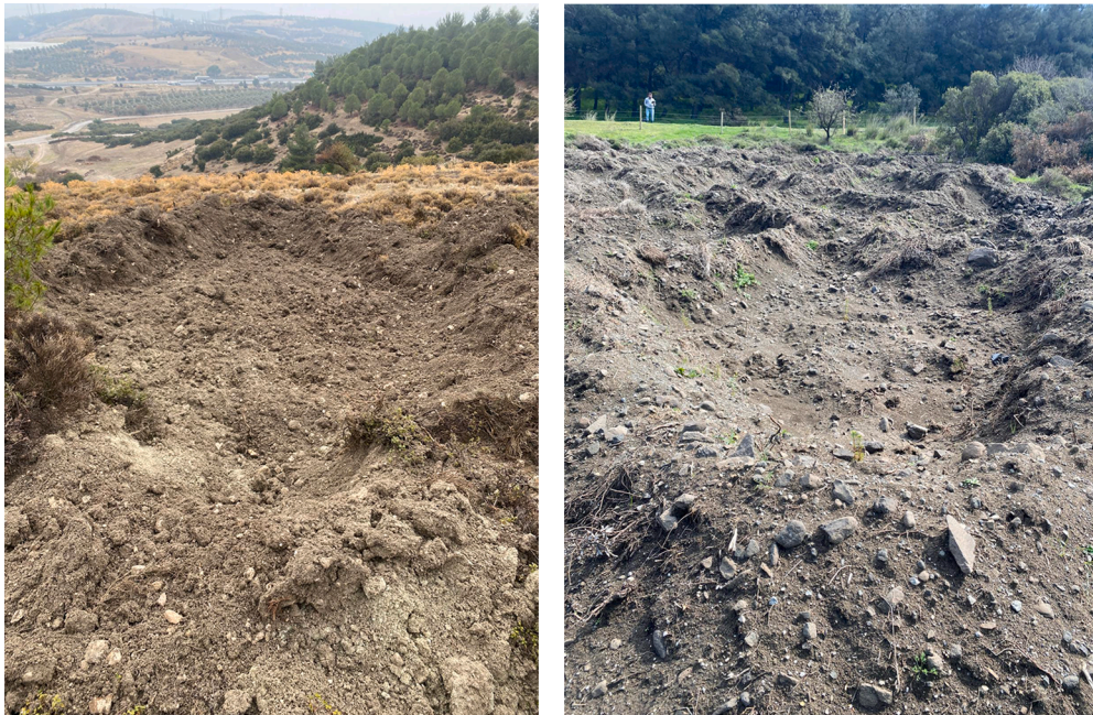
Figure 6.8 Constructing a diamond-shaped microcatchment in Izmir, Türkiye. (Photo: Muhammed Ali Aydin) Study in Türkiye are examining different shaped microcatchments to increase water retention (Esen et al., 2024).
