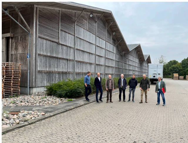
Figure 10.3 More than 25-years-old wooden industrial buildings (9500 m 2 ) built in 1995 at the Velux company's production facility in Østbirk, Denmark, to demonstrate a sustainable solution in practice to the alternative of using energy-intensive construction materials like concrete, aluminum, steel, and plastics. Specifications for the buildings included the use of proactive construction solutions to avoid the need for paint or chemical treatments to support durability, to avoid the need for maintenance, and to support aesthetics and functionality of the building. (Credit: Palle Madsen.)
