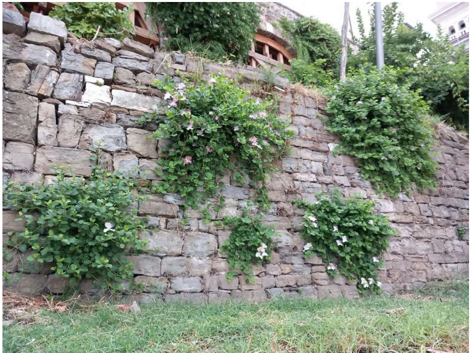
Figure 2: Proposed renovation of terraced landscape: Dry stone wall with vegetation (Capparis spinosa) supporting the sloped terraces. Image Credit: Cécil Meulenberg.
