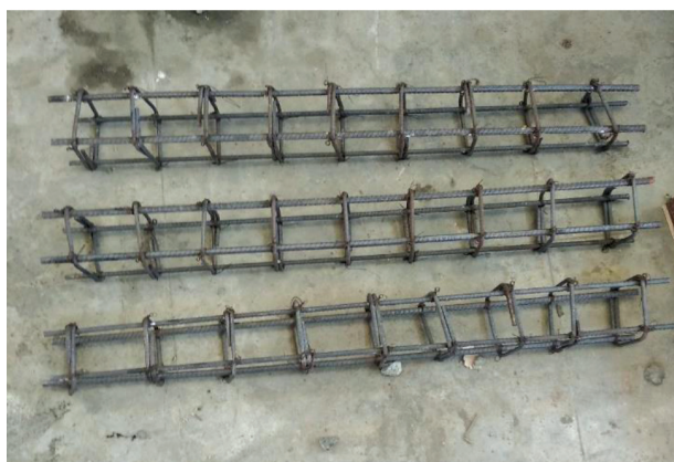
Figure 3: Reinforcement details and casting of a beam
