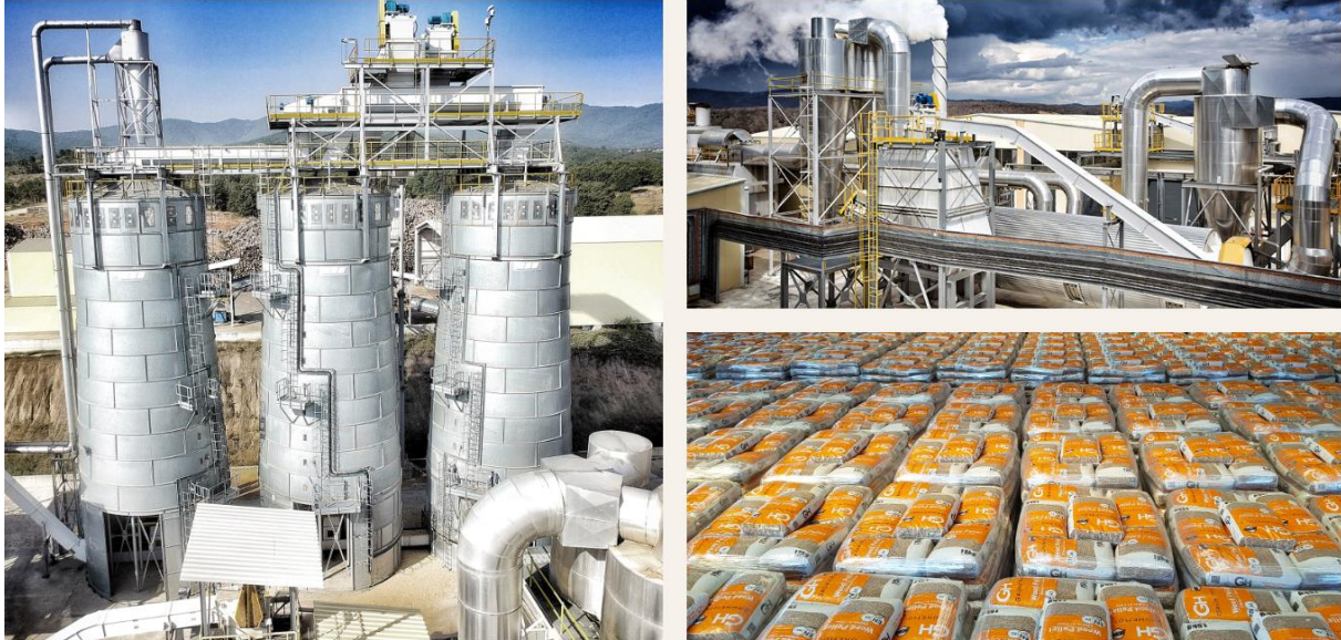
The industrial facilities of Alfa Wood Group in Nevrokopi-Drama
