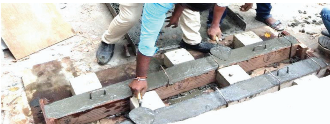
Figure 4: Beam Casting
