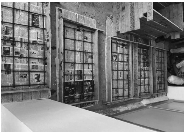
Figure 3: Placing of the reinforcement in the mould
