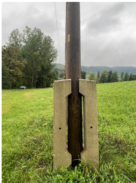
Fig. 2: Double A-type pole (left) and installation of single N-type poles into concrete clamps (right)
