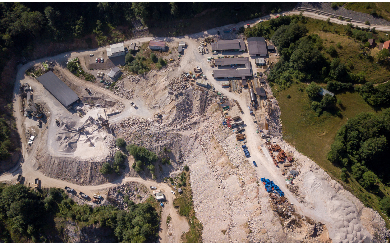
The impacts of the Ulog dam construction become impressively clear when flying a drone. Photos: Vladimir Tadić
