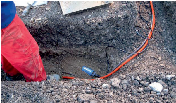
Figure 3. Installation of TDR probe.
