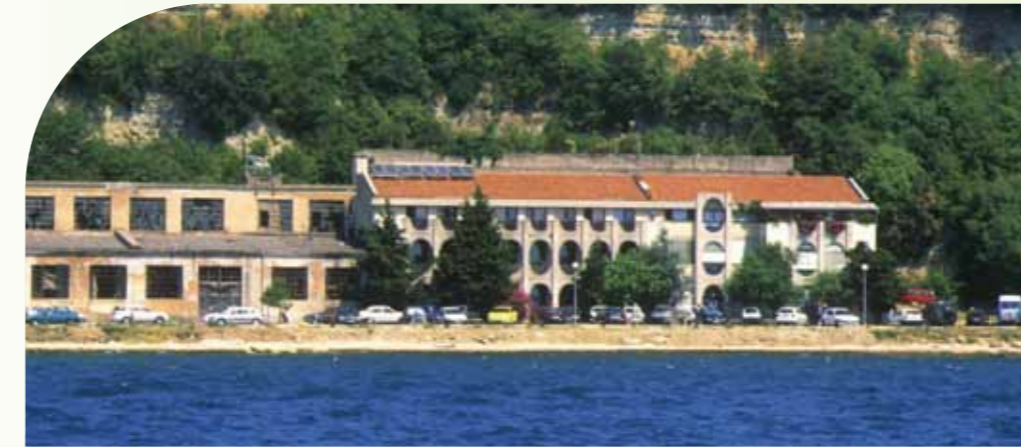
MBP v prostorih tovarne Salvetti v Fornačah v Piranu / MBS in the premises of Salvetti Factory in Fornače in Piran (1980 - 2004)
