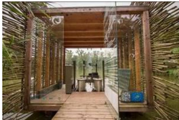
Figure 9: Completed wharf at Koseze Pond
