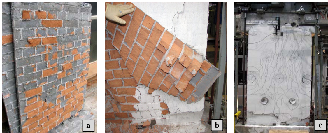
Fig. 6. Coating separated from the wall (a), delamination of epoxy based coating (b) and failure of anchors at highest density (c).
