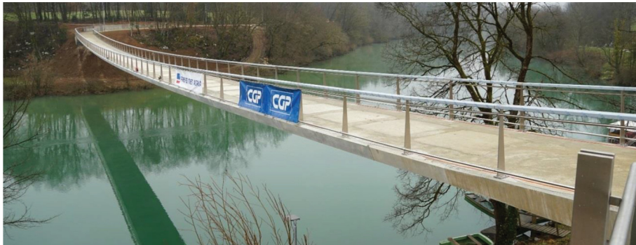
Figure 1. Bridge on the day of the diagnostic load test.
