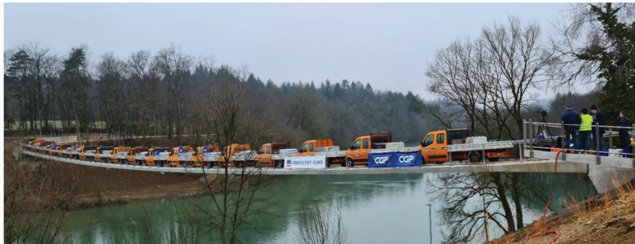
Figure 4. In the static load test (Phase 2), all 18 trucks with an overall 70.4 tonnes were present on the bridge.
