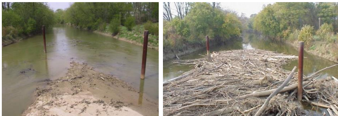
Figure 35: Debris deflectors (cylindrical vertical structures) without and with debris, respectively (modified from (Dennis A. Lyn, Thomas Cooper, Yong-Kon Yi, and Sinha 2003))
