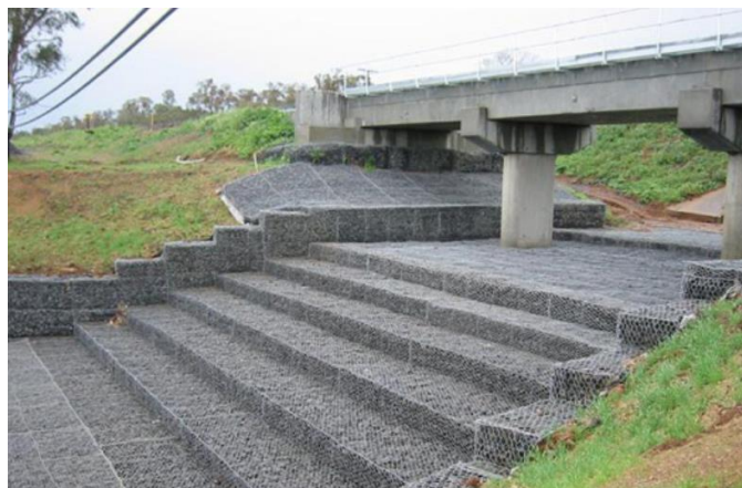
Figure 30: Example of a gabion mattress installation (Gabionet Environment Solution 2014).
