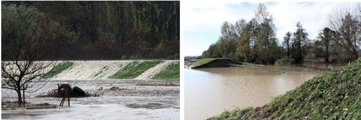
Figure 1: Overtopping (left) and breaching (right) of a flood protection embankment Virje – Otok Brezje in north Croatia in 2012., from Bačić et al. (2017)
