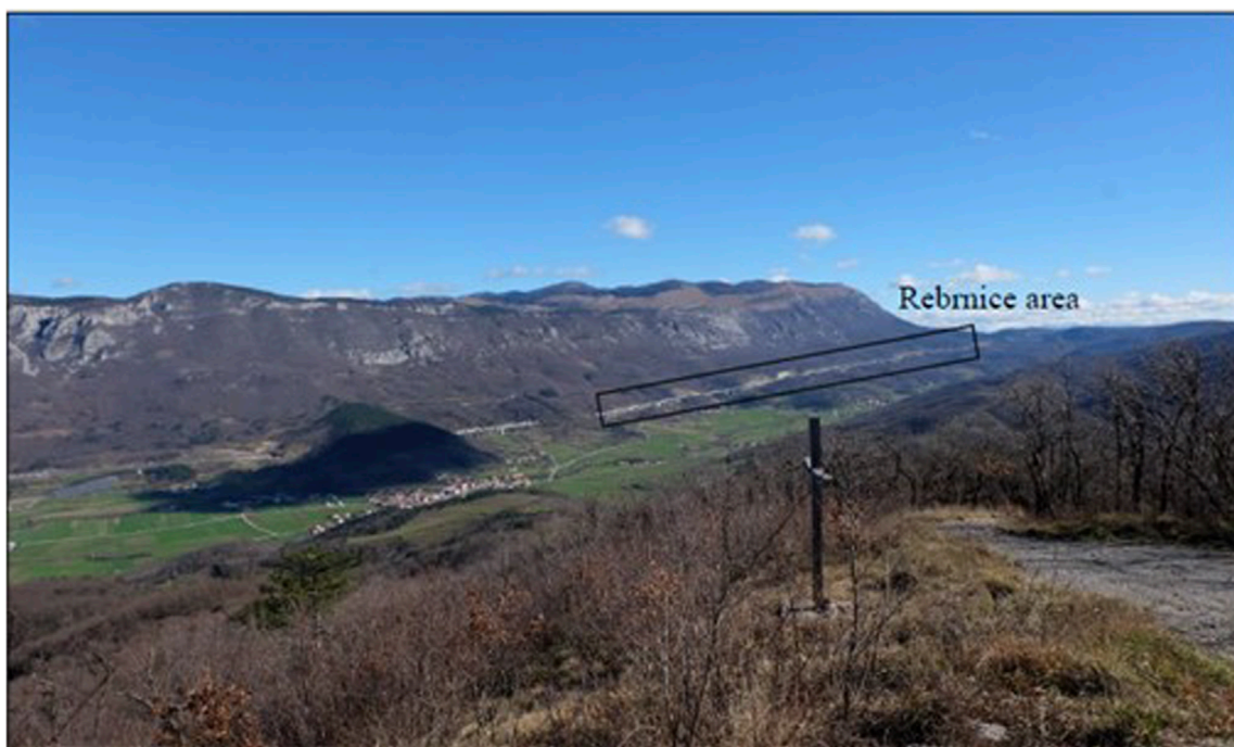
FIGURE 8 Rebrnice area and the motorway in the Upper Vipava Valley.
