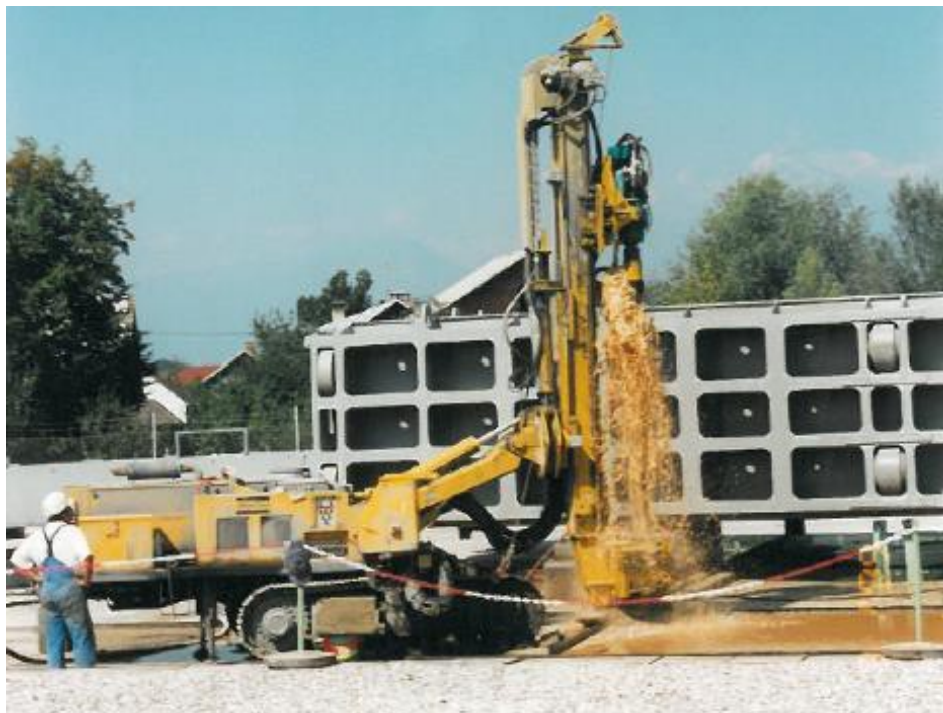
Fig. 8 Rehabilitation works at the right bank of the dam
