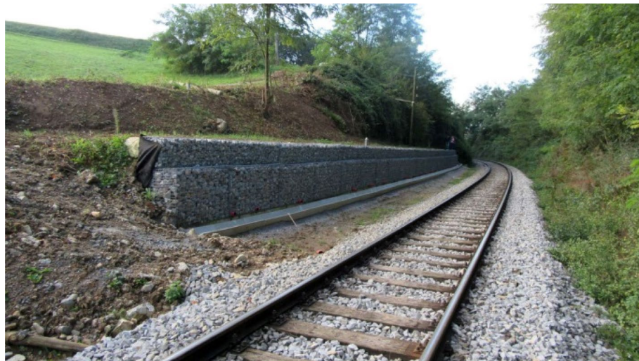
Figure 14. Picture of the retaining wall structure.
