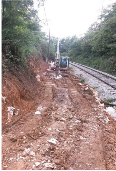
Figure 4. Location of the large demo structure.
