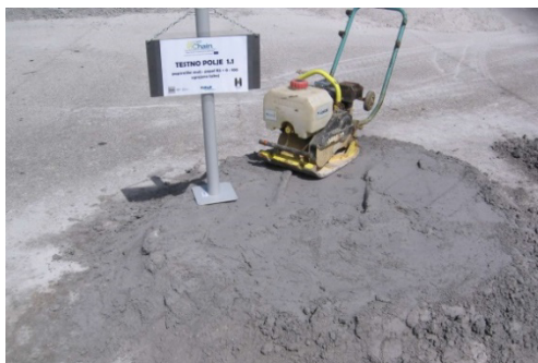
Figure 1: One of the test fields with the compactor.
