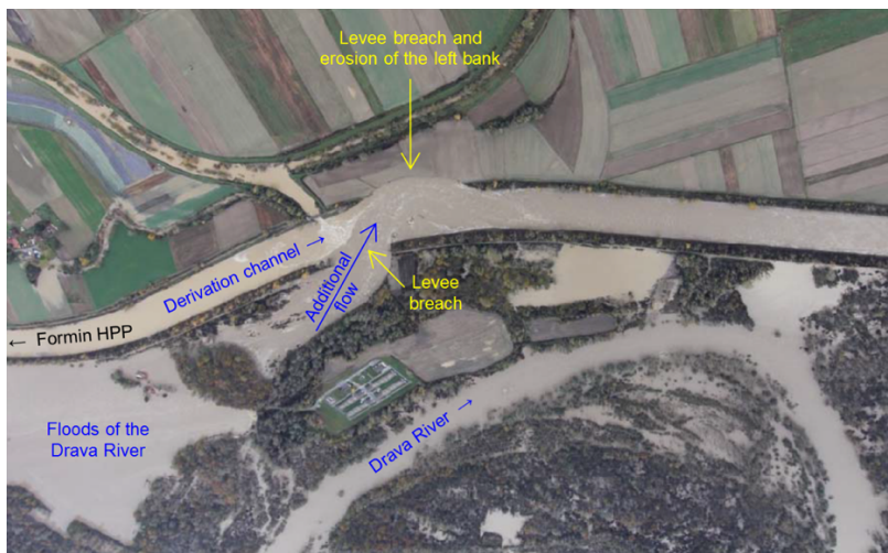
Fig. 12. The area with the greatest damage - during flooding (Photo: Mensuras photo archive).
