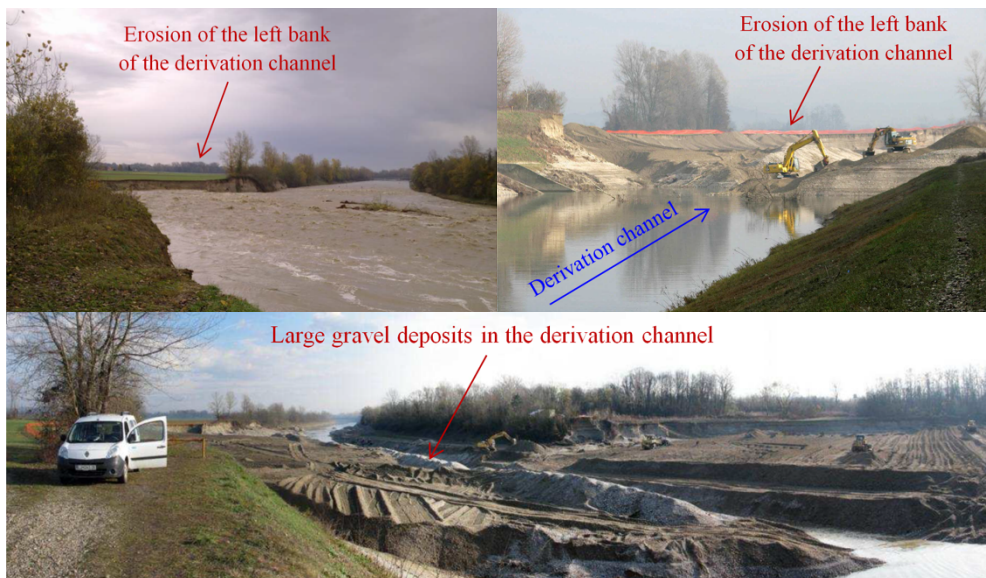
Fig. 14. Erosion of the left bank of the derivation channel and large gravel deposits in the derivation channel (Photos: DEM photo archive and A. Geršak).
