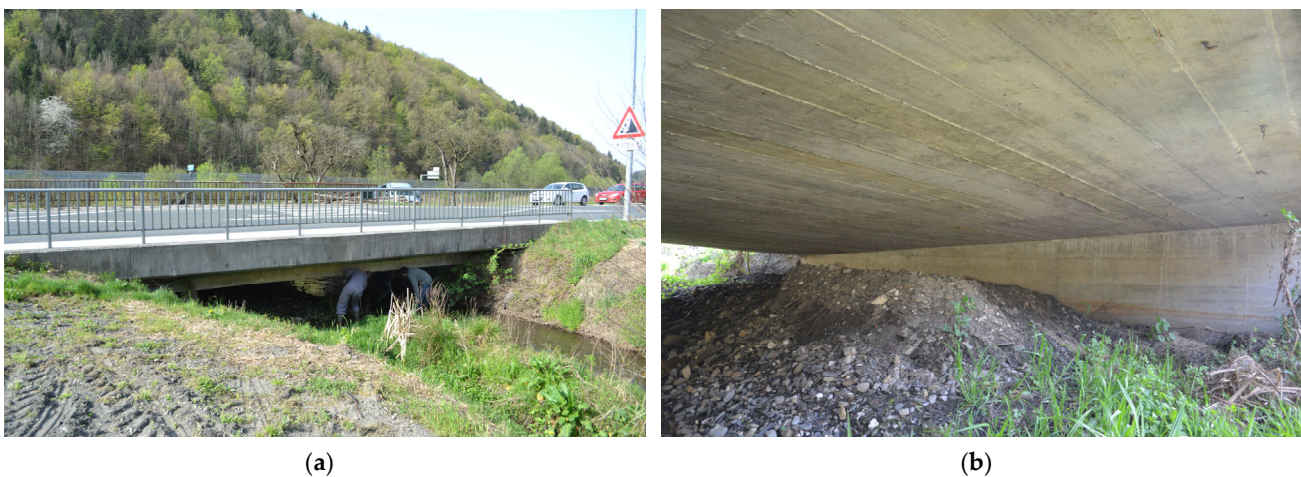
Figure 5. Test bridge. (a) Side view; (b) under the bridge.
