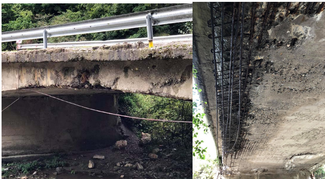
Figure 1. Reinforced Concrete Bridge in Drelaj-Peja –photo (25.12.2018)
