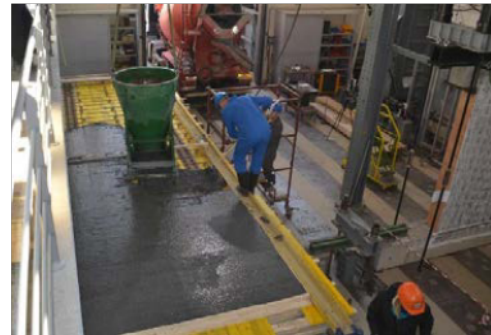
Figure 4: Strengthening process of the steel bridge
