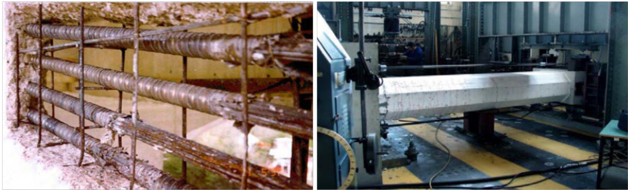
Figure 3: Corrosion of prestressed I-shaped beam in 1996 (left) [6] and experimental studies of scaled bridge pier (right)
