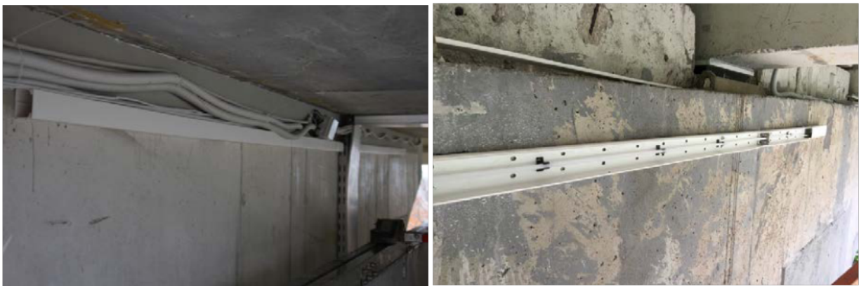
Figure 12: Smartec SOFO sensor, installed at the side of the pier cap on the left viaduct: covered (a) and uncovered (b)
