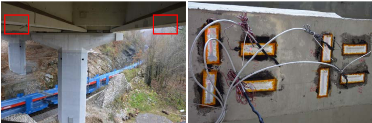
Figure 5: Two strain gauge locations on external and internal beams of the right viaduct – marked with red line (left) and 4 strain gauge sensors, all mounted at the same location on external beam of the left viaduct (right)
