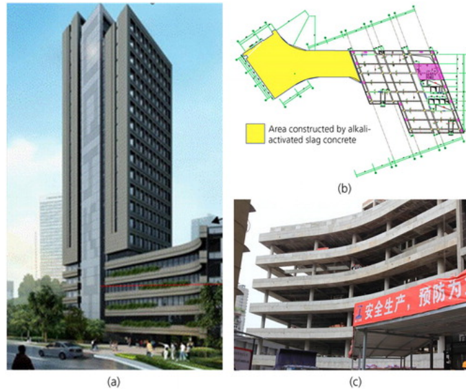
Fig 3: Illustration of the alkali-activated slag demonstration project: (a) effect drawing of Jianke Chongqing; (b) illustration of the construction section; (c) side view of the structure made with alkali-activated slag concrete
