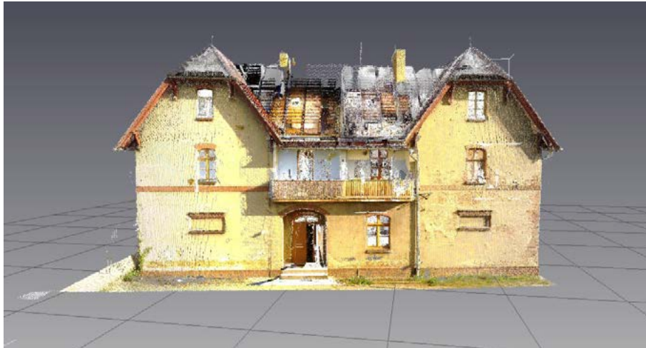
Figure 2: Point cloud of the house
