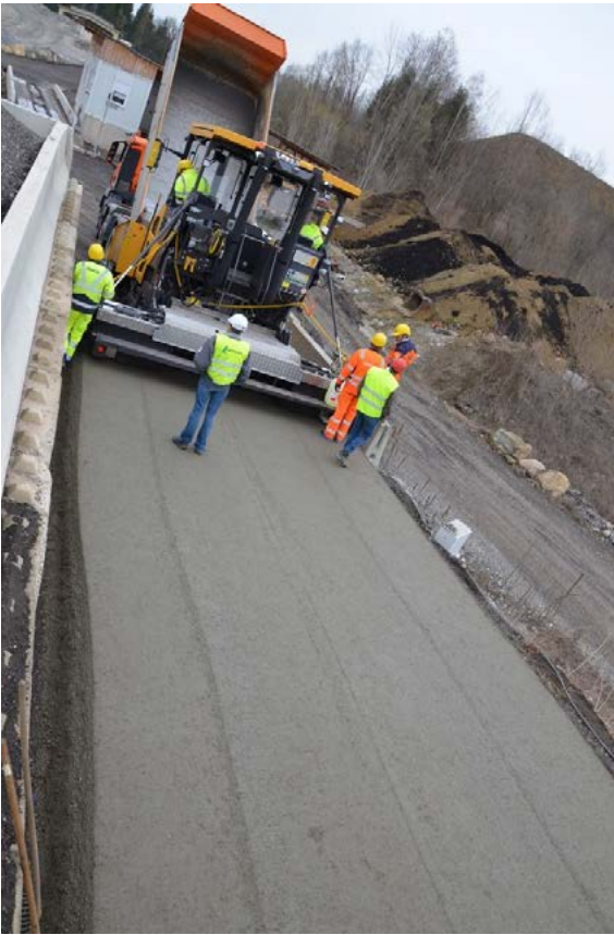
Figure 4: Placing concrete with asphalt paver
