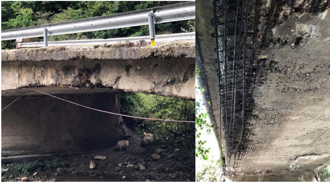
Figure 1. Reinforced Concrete Bridge in Drelaj-Peja –photo (25.12.2018)
