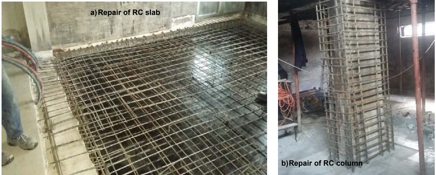
Figure 12: Repair of: a) RC slab, b) RC column
