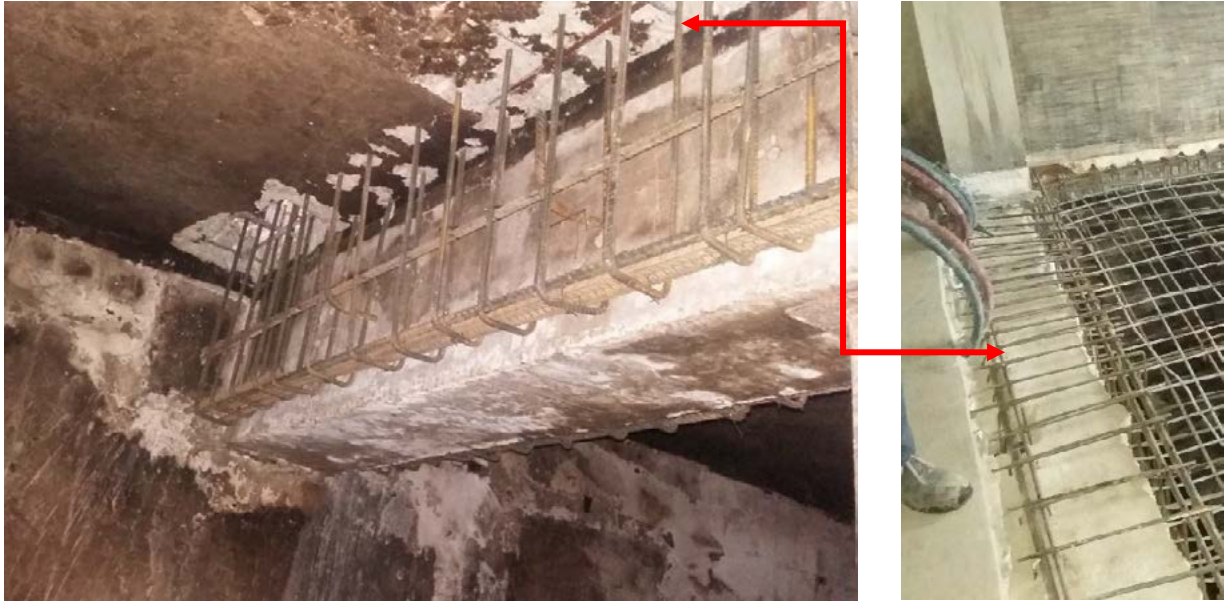
Figure 14: Repair of RC beams
