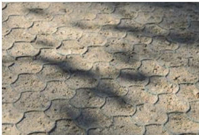
Figure 5. Geocells in pavement structure before asphalt laying
