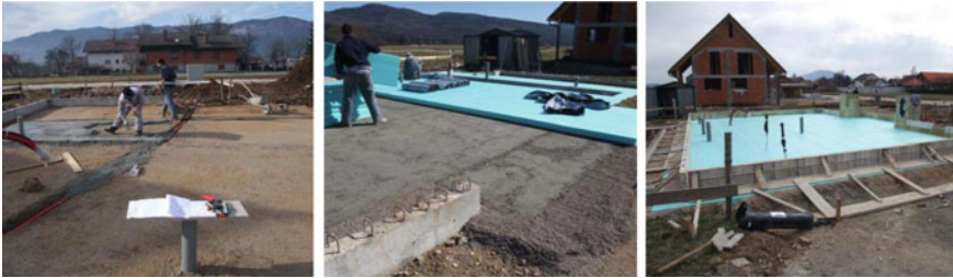
Fig. 3.3 Example of extruded polystyrene (XPS) insulation boards used under the foundation slab. Source Summarised from Fibran (2020)
