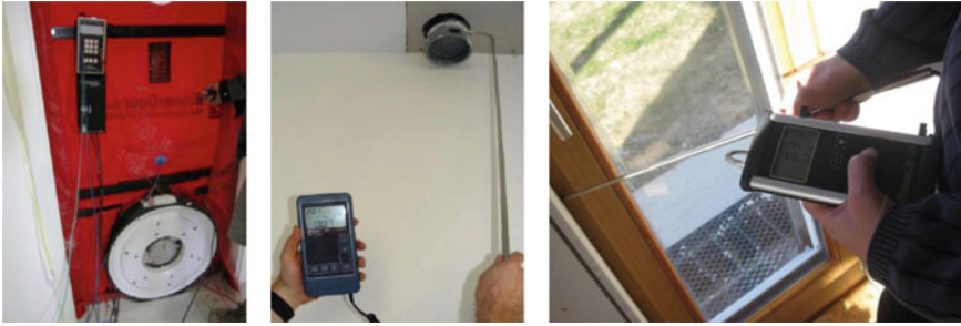
Fig. 4.1 Investigations of the building envelope airtightness: in search of leakages with a handheld anemometer. Source Building and Civil Engineering Institute ZRMK (authors: Praznik, M. and Malovrh, M.)
