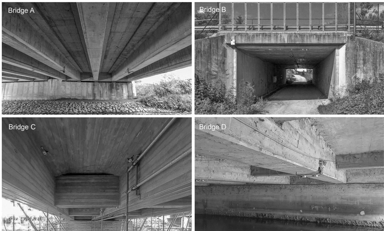
Fig. 8 The four test bridges
