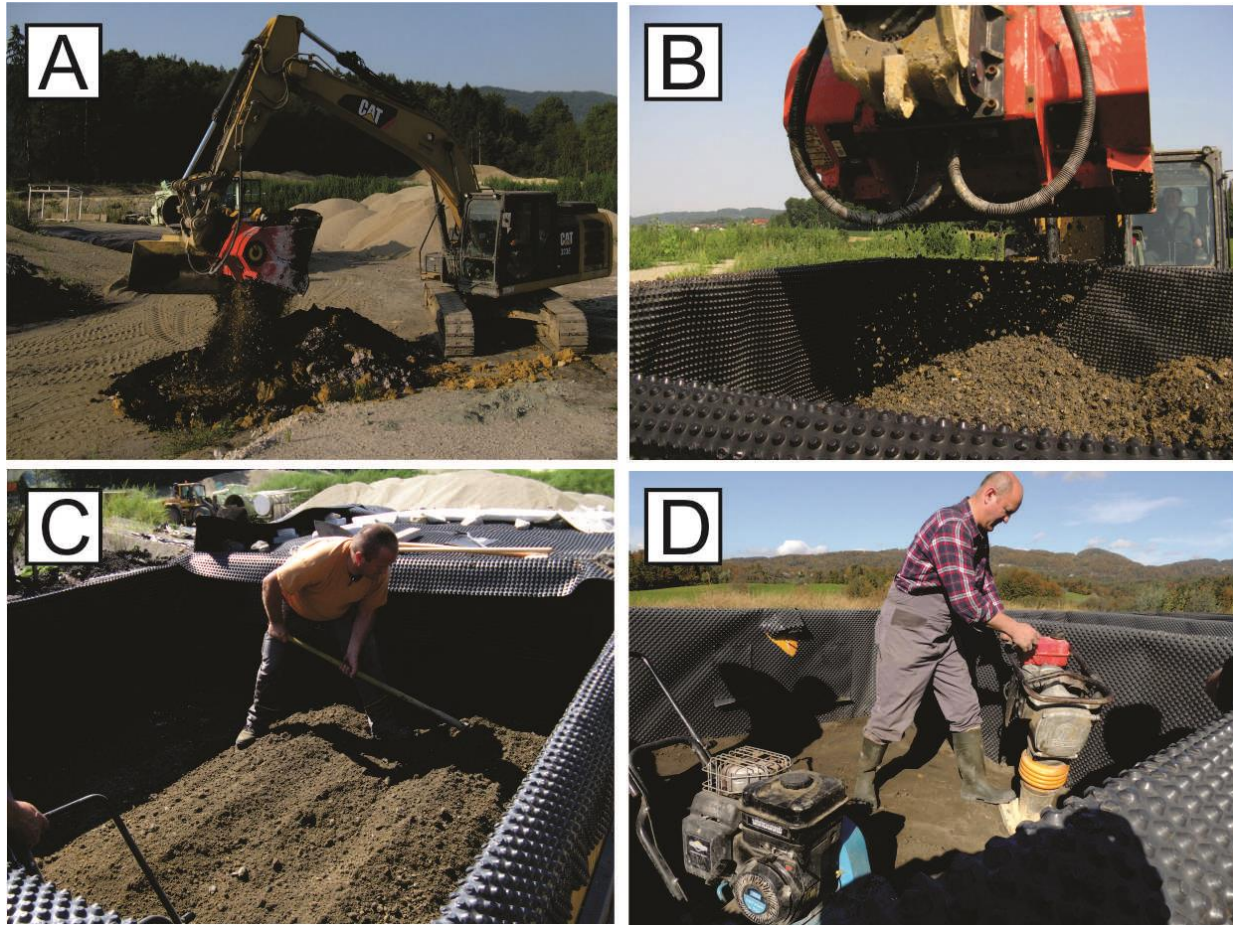
Figure s3 Different stages of a field preparation of geotechnical composites for the lysimeter experiments: Preparation of a composite, according to predetermined dry mass ratios and with addition of optimal amount of water, by the use of excavator mixing bucket (A), filling of the lysimeter with a layer of a composite (B), spreading of a composite in a layer of uniform thickness of 30 cm (C), and the final installation of the layer of a composite by a vibration compactor in box lysimeters (D).
