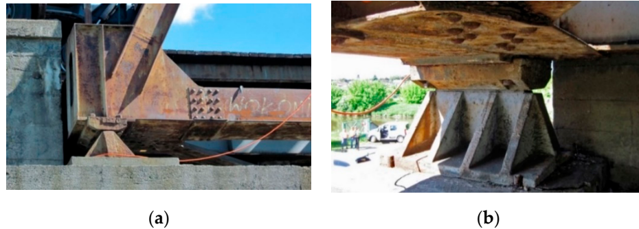
Figure 5. Nieporeć Bridge bearing (a). edge and (b). view from underneath bridge.
