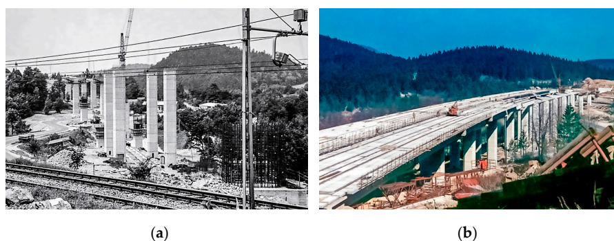
Figure 1. Construction of the (a) Piers [25] and (b) Superstructure [26].
