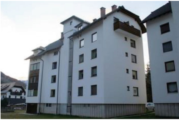
Fig. 3 Reference building, a typical residential building from the period 1971–1980
