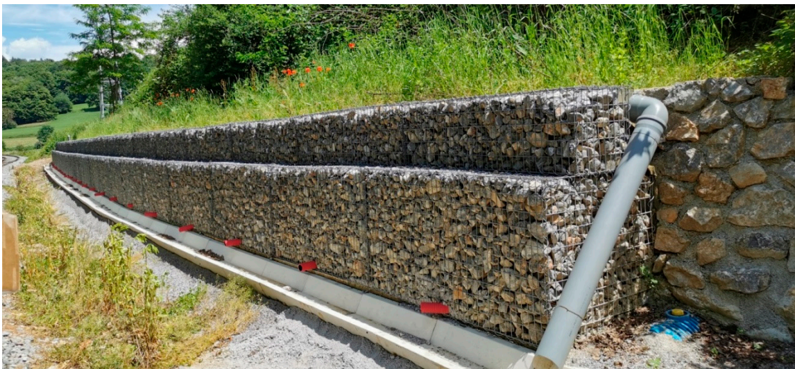
Figure 11. Retaining wall with gabions and the composite as the backfill material.
