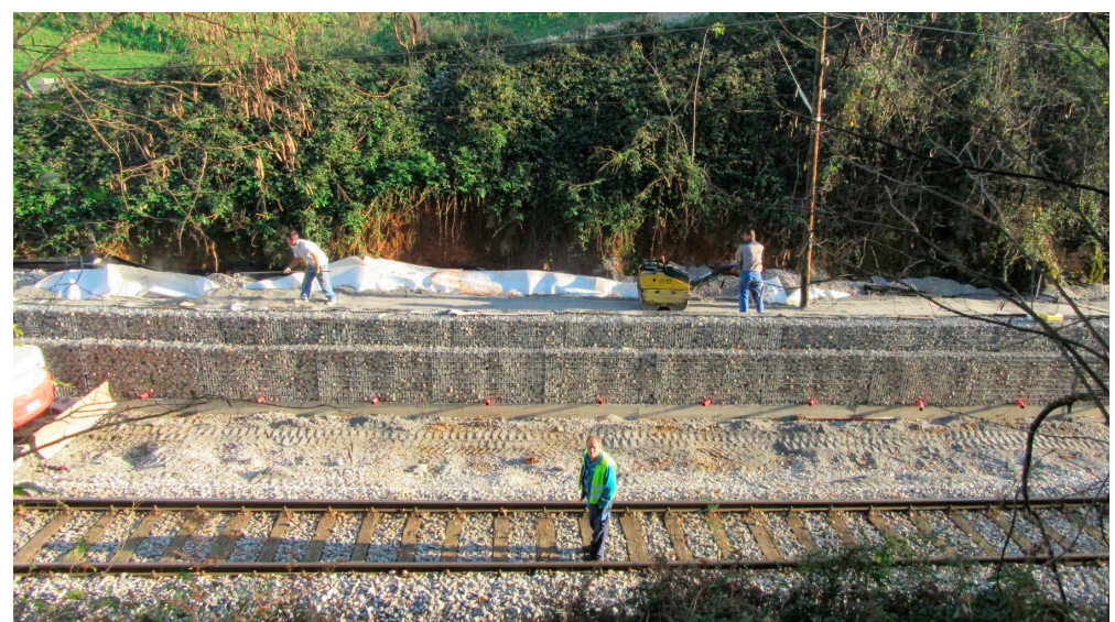
Figure 3. Compacting the last layer of the composite.
