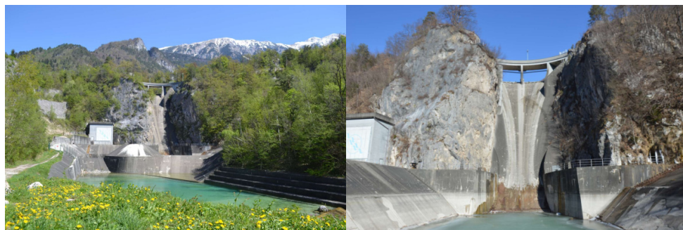
Figure 4. Distant and closer view of the Moste Dam from the downstream side (Photos: P. Žvanut).
