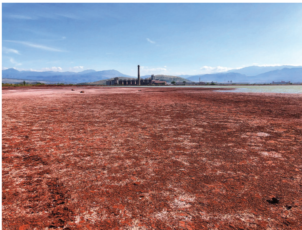
Figure 7. Red mud - bauxite residue tailings dams, Podgorica.
