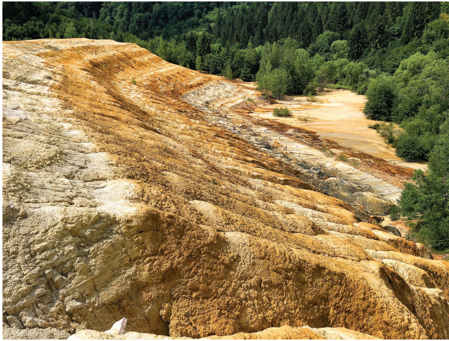
Figure 8. Flotation tailings dam at "Gradac".
