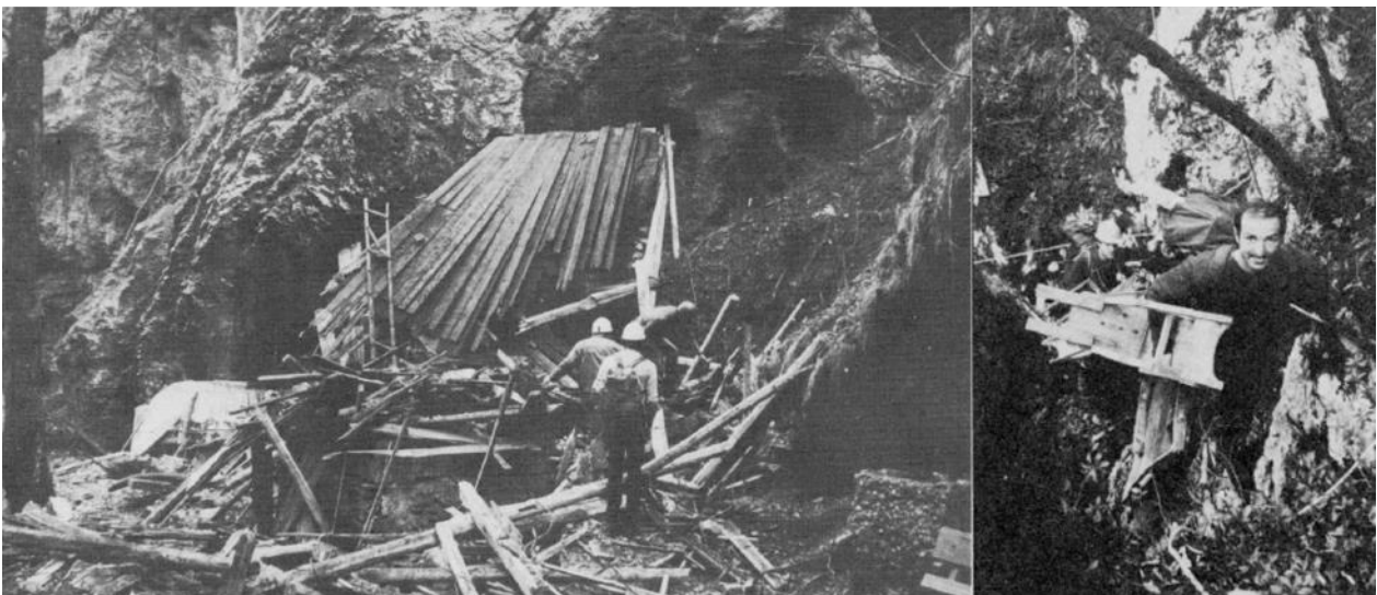
Figure 52 Demolished barracks (left) and an alpinist rescuing exhibits after the rockfall (right)
