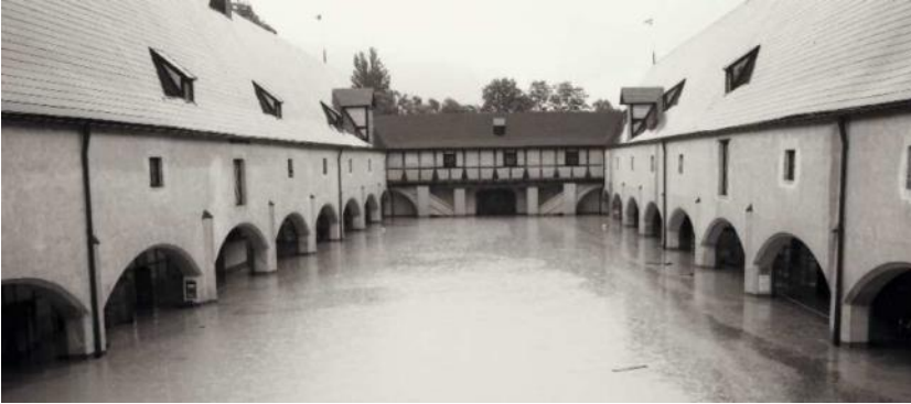
Figure 56 Flooded Zeughaus in 1985(© M.Pizzinini)
