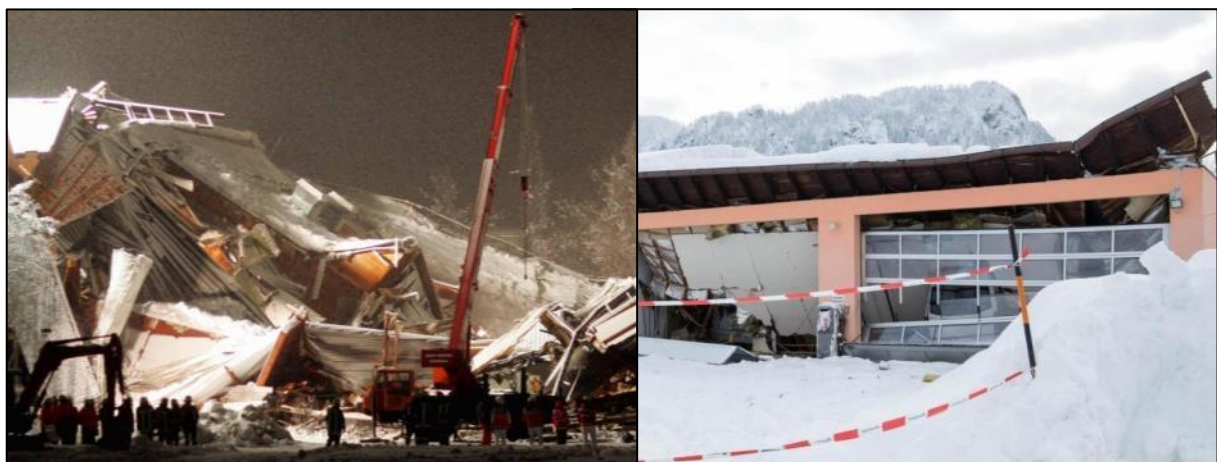
Figure 49 Lack of maintenance and bad construction as a reason for the collapse of the ice stadium in Bad Reichenhall, 2006 and collapse of a small barn less than 15km from the Glockenbachschmiede, 2019/01/11
